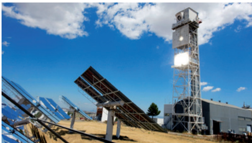
Fig. 72: Facility for testing the receiver systems (Source: DLR/Ernsting)
